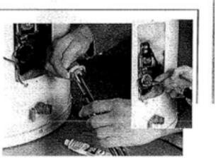
Coat the element's threads and rubber washer with pipe joint compound, and screw the element in place.
