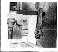
Test the T&P valve periodically (inset), and remove it if it seizes up or cloesn't seem to work properly.
