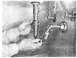
To remove a sink basin drain, loosen the two P-trap nuts and remove the trap. Keep a bucket under the trap to catch waste water.
