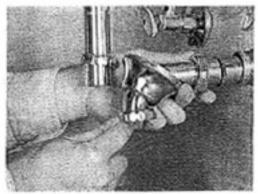
To remove the P-trap arm, disconnect the friction nut at the wall and pull the arm straight out from the drainpipe.
