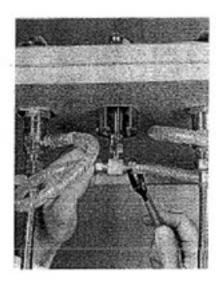
To remove a bottommounted faucet, undo the connecting tubing and remove the jamb nuts.
