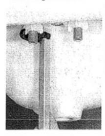
To remove a topmounted faucet, use a basin wrench to unscrew the jamb nuts from the faucet sharks.
