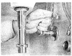
3 To disconnect the sink drain's pop-up linkage, squeeze the tension clip and slide the clevis from the lever.
