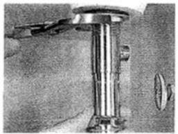
4 Use groove-joint pliers to loosen the nut that holds the sink drain in place. Backhold the drain with a second pair of pliers if it spins.
