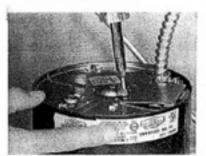
Once you have disconnected the disposal unit, lower it and turn it over. Use a screwdriver to remove the electrical bex sever.
