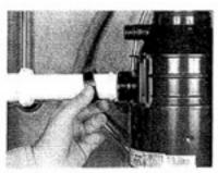
Remove the waste connection at the side of the disposal unit. Some are bolted in, and some have a compression nut.
