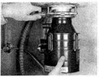
3 Insert a screwdriver into one of the tabs of the retaining ring as shown, and rotate the ring counter clockwise.
