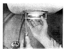
7 To remove the waste disposal unit drain fitting from under the sink, loosen the three bolts in the retaining ring.
