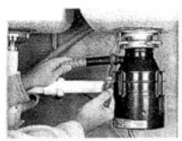
Unscrew the hose clamp on the dishwasher discharge hose. Pull the hose from the disposal unit's infet nipple.
