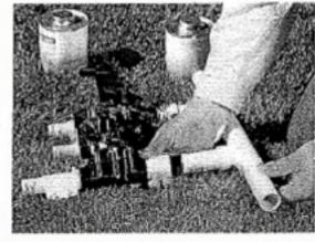
1 Following the layout of your system, assemble the zone valve piping above ground so that you will have room to work.
