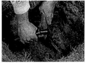
Use a scissor-style pipe cutter to slice through polyethylene pipe. Push the pipe into the fittings until they bottom out on the barbs.
