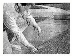
Install the grit strainers and nozzles on the sprinkler heads, and adjust the heads for the best coverage.
