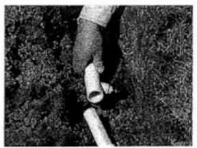
To drain a supply line low point, install a T-fitting with a threaded branch. Screw a brass drain into the branch.
